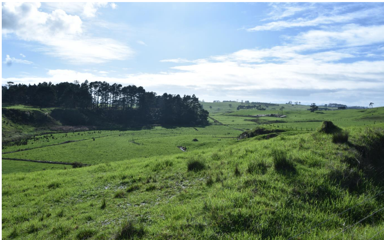
Figure 4. A downstream north-east view from the right abutment
