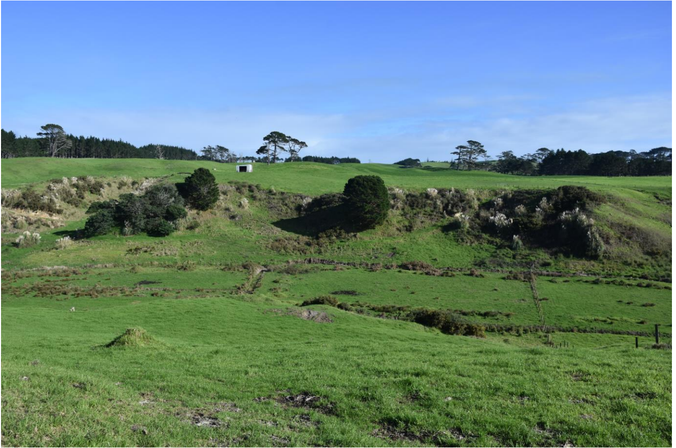
Figure 5. Photo of the stream channels at the approximate site of the proposed embankment (looking west).
